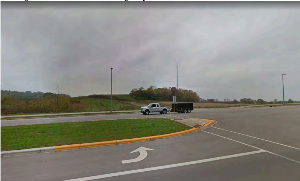
Looking west from Junction Road/Highway M toward Temin Trail turn
