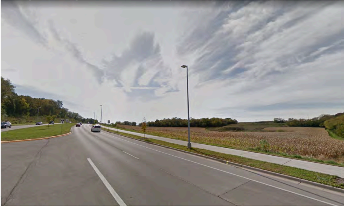
Looking south along Junction Road/Highway M
